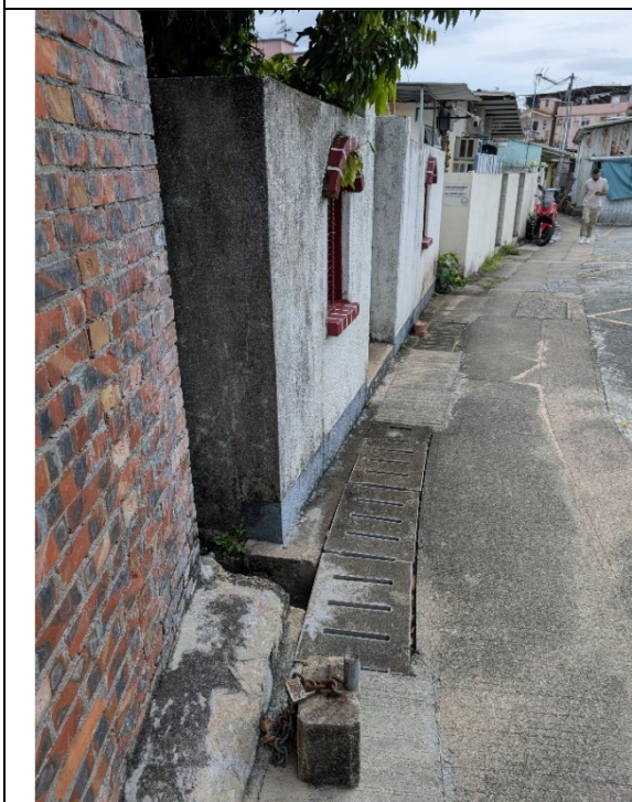
Plate 9 – Existing 375mm channel at the downstream of the northeast corner of the Application Site flowing to the north.
