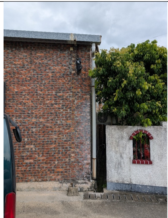
Plate 8 – Existing 225mm channel running along the northern boundary of the Application Site with existing gutter at the roof edge discharging into the existing channel.
