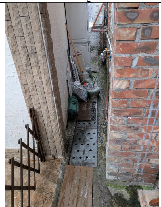
Plate 10 – Existing 225mm channel between the existing main building and the associated small building at the northwest corner of the Application Site.
