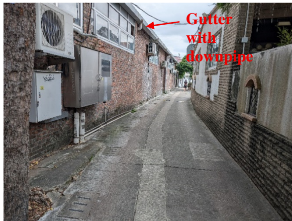
Plate 5 – Existing 225mm channel running along the eastern boundary of the Application Site flowing to the north. Existing gutter at the roof edge of the ‘Red Brick House’ with downpipes discharge into the existing channel.
